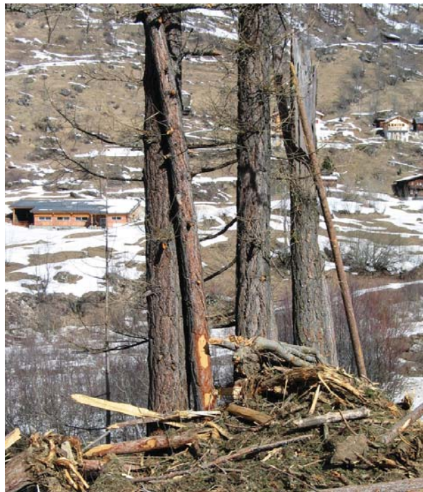
Avalanche damage in the Swiss Lötschental valley.
